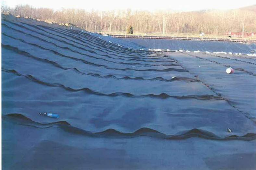
Photo 14 - Deployment of geocomposite drainage layer along the south slope
