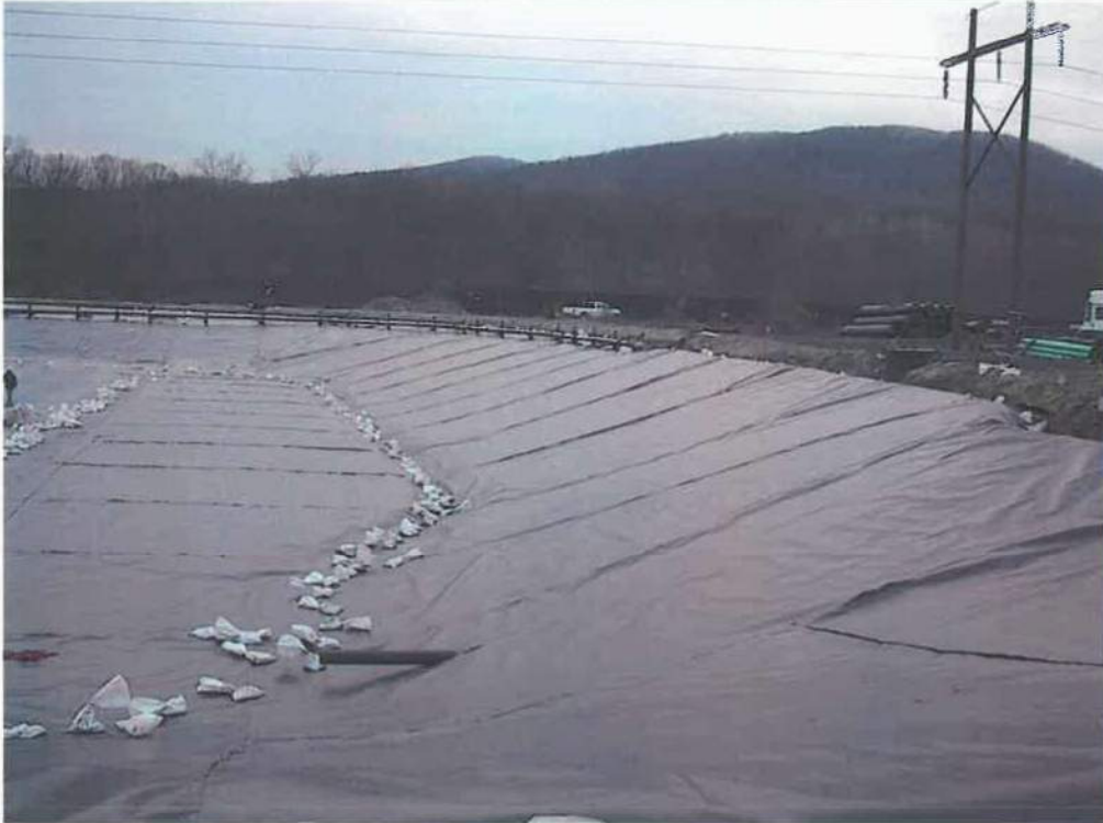
Photo 11 - Deployed and seamed 40 Mil HDPE liner along the north slope
