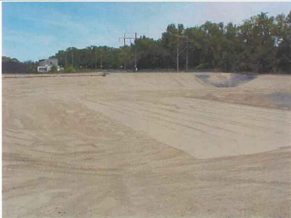
Photo 6 - 6" sand bedding over the entire basin
