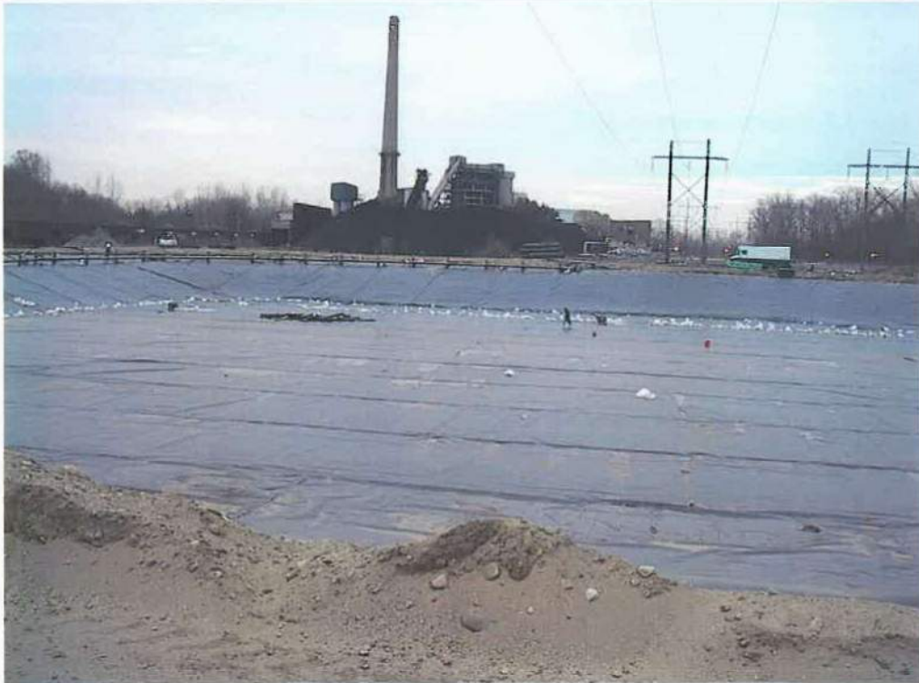
Photo 13 - Completed 40 Mil HDPE liner viewing from the south to the north
