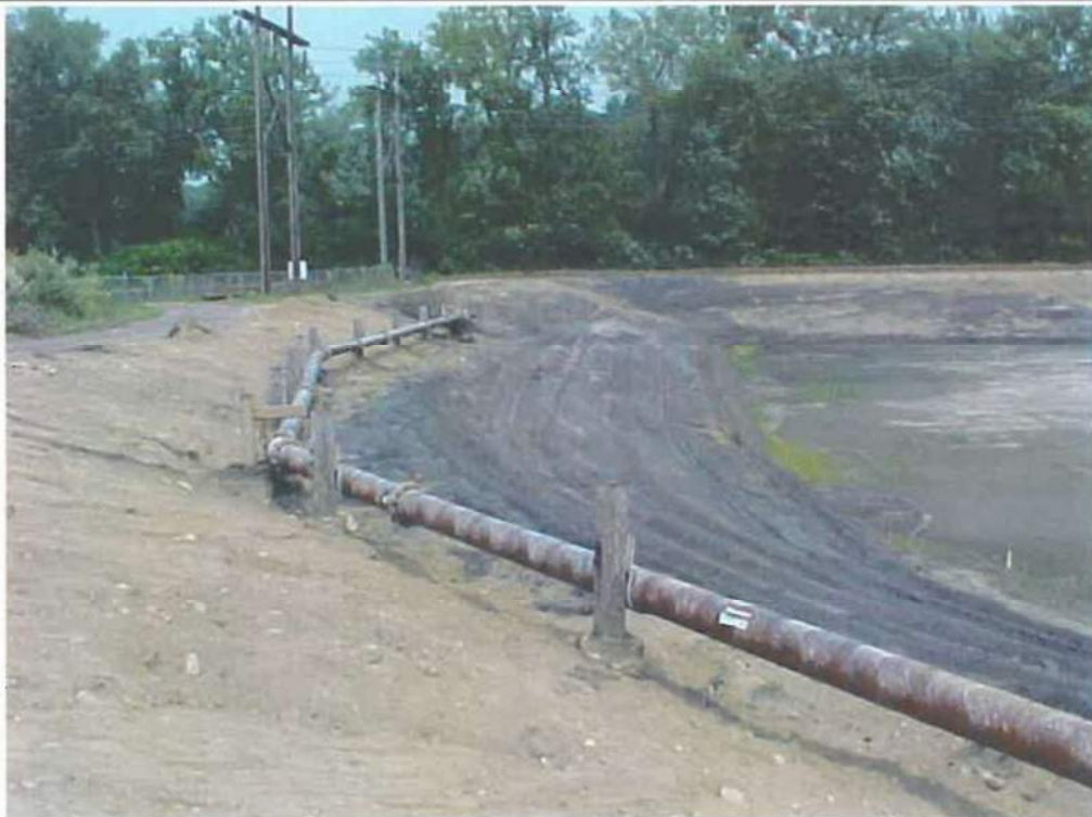
Photo 2 - Pre construction conditions of the north slope
