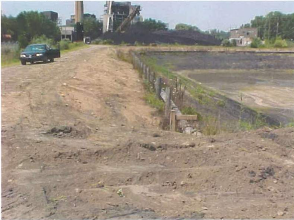
Photo 3 - Pre-construction conditions along the west slope
