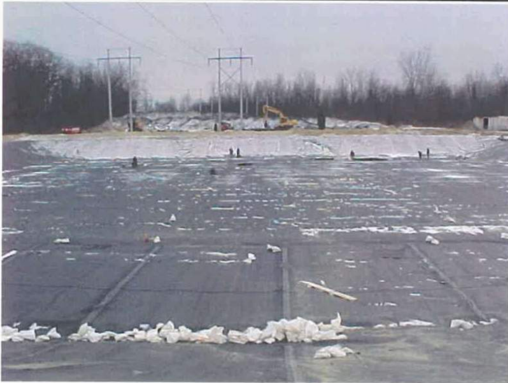
Photo 18 - Completed 60 Mil HDPE liner viewing from north to south
