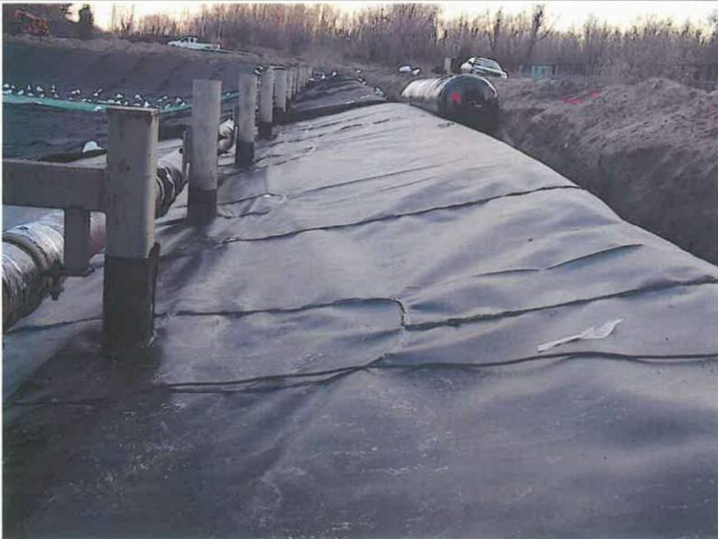
Photo 12 - Typical 40 Mil boots along the top of the west slope
