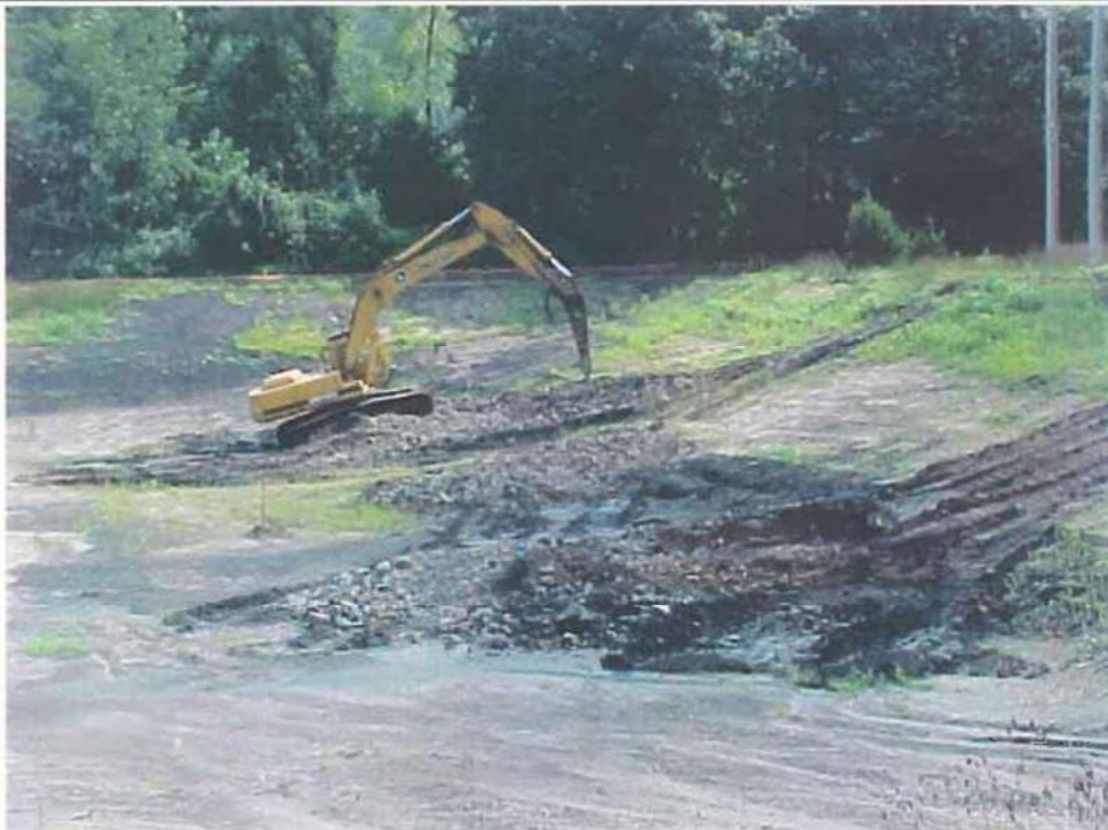
Photo 4 - Site preparation of the south slope
