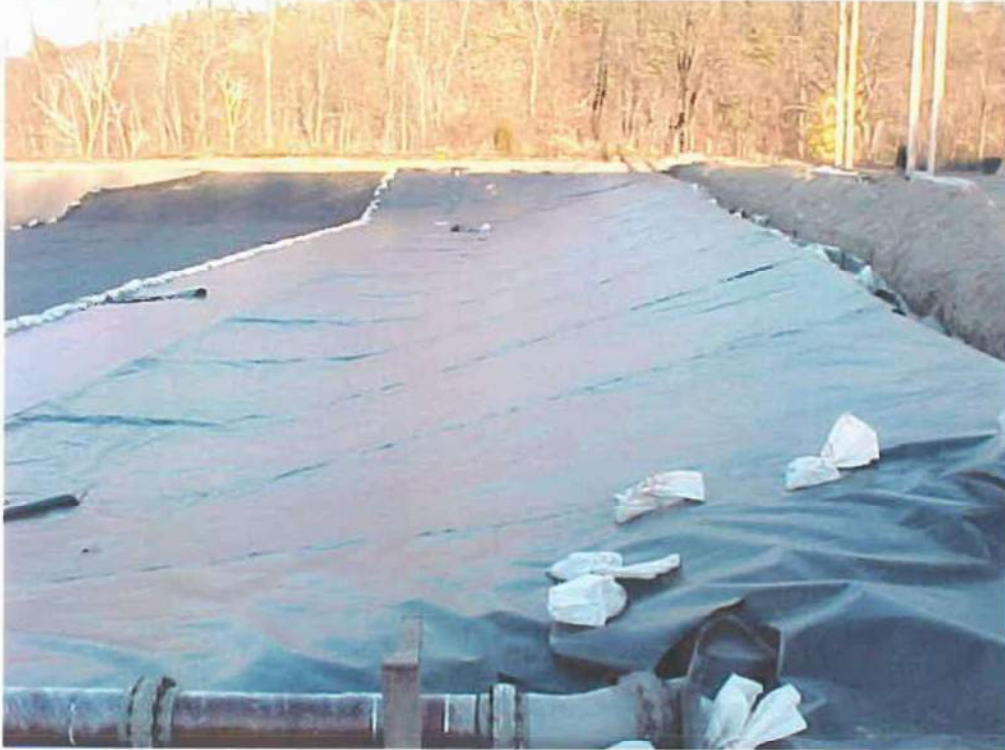
Photo 9 - 40 Mil HDPE liner deployed and seamed along the south slope
