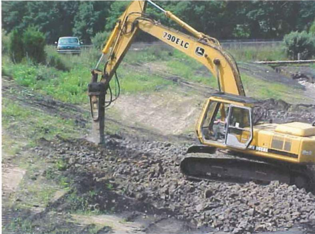
Photo 5 - Ledge removal along the south slope
