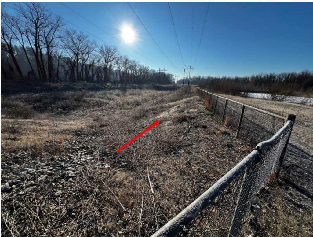
Photo 4 – Interior slope of west embankment looking south; note area of marginal vegetation (red arrow) and riprap in lower left of photo
