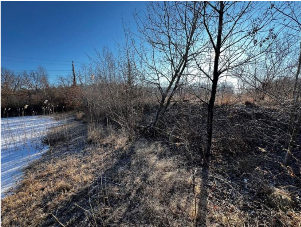
Photo 25 – North exterior slope along coal pile sump; note woody vegetation
