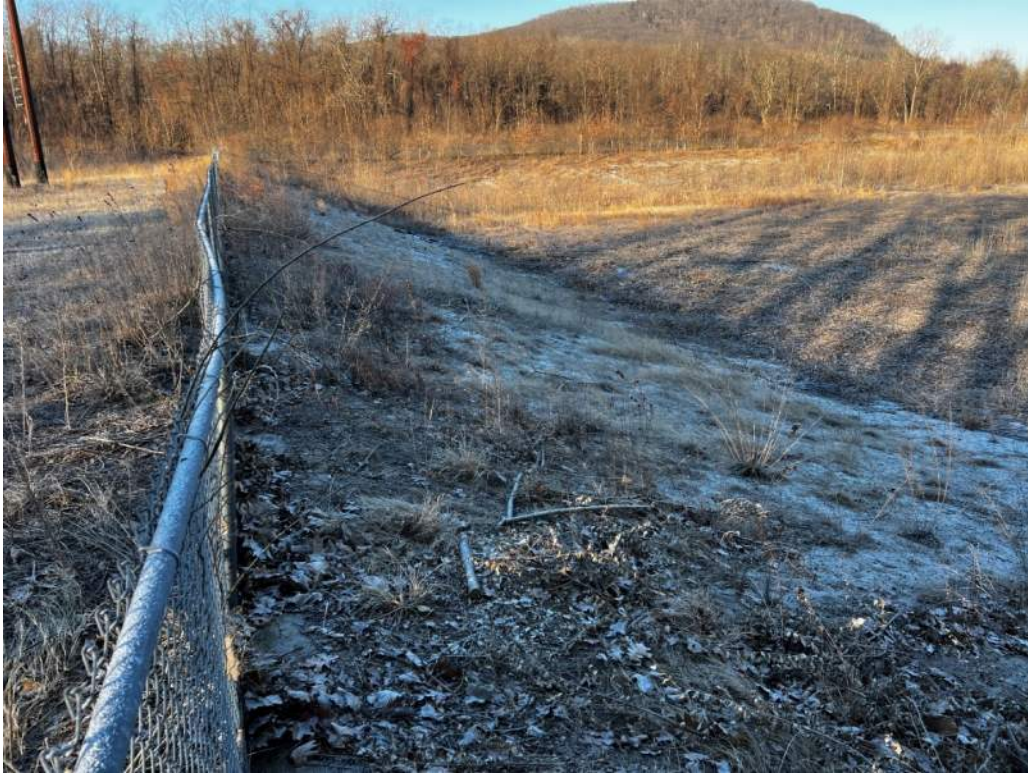
Photo 13 – South interior slope; note marginal vegetation
