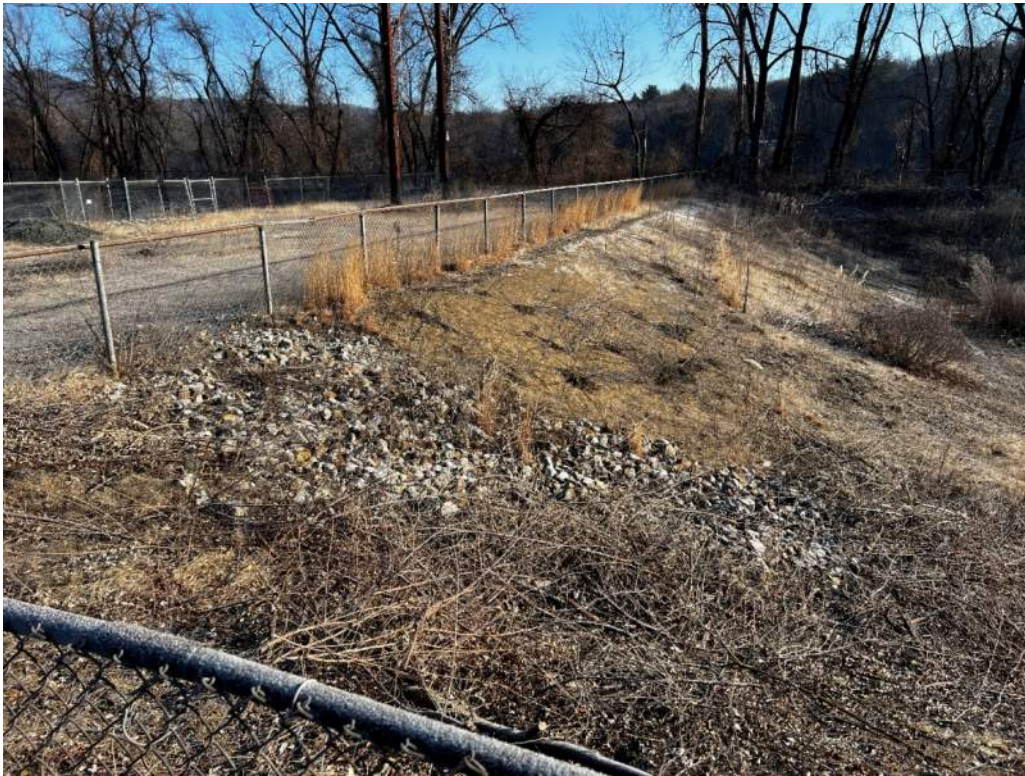
Photo 9 – Interior slope of north embankment; note riprap on slope and sparse vegetation
