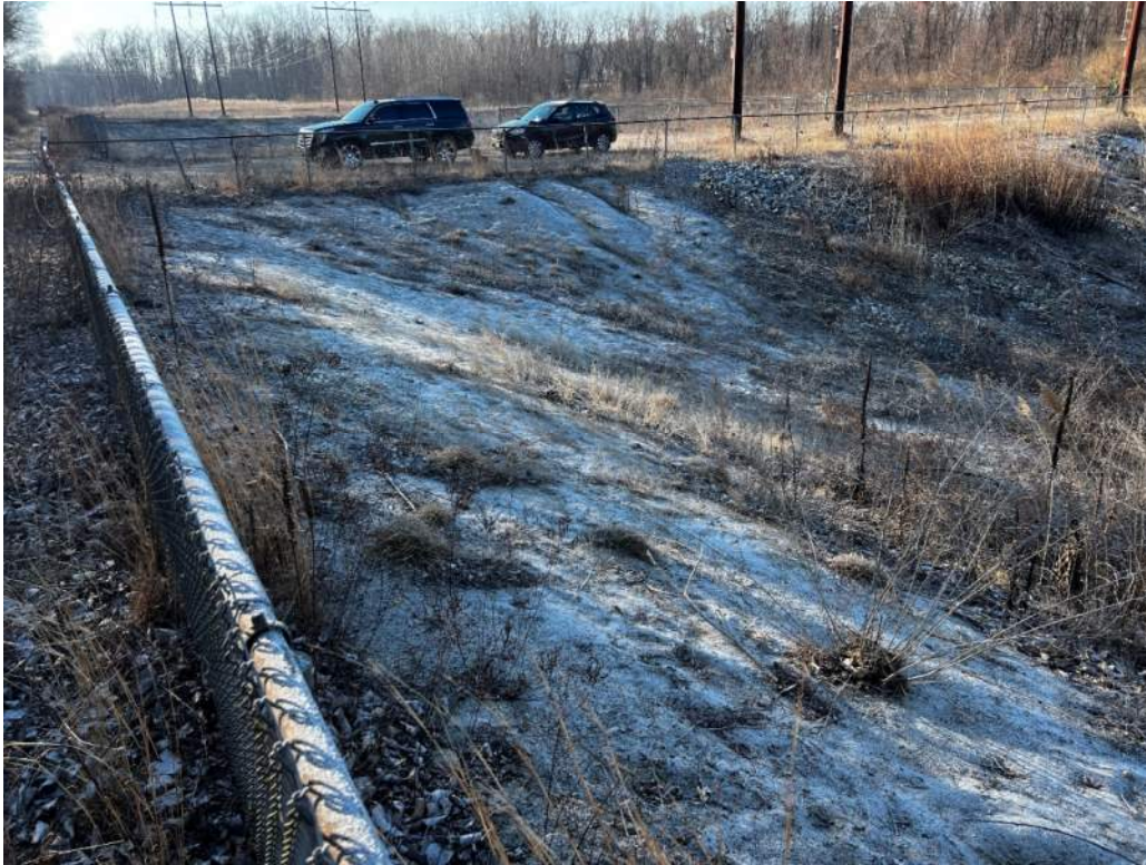
Photo 17 – Junction of east interior slope and south interior slope; note marginal vegetative cover and erosion rills
