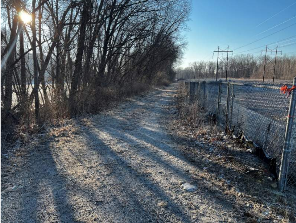
Photo 3 – Crest of east embankment; note sparse vegetation and minor rutting
