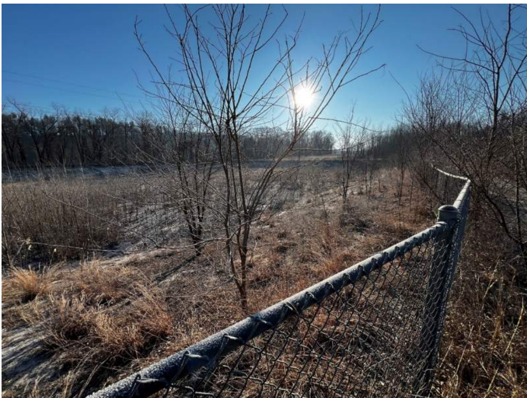
Photo 22 – West interior slope; note woody vegetation
