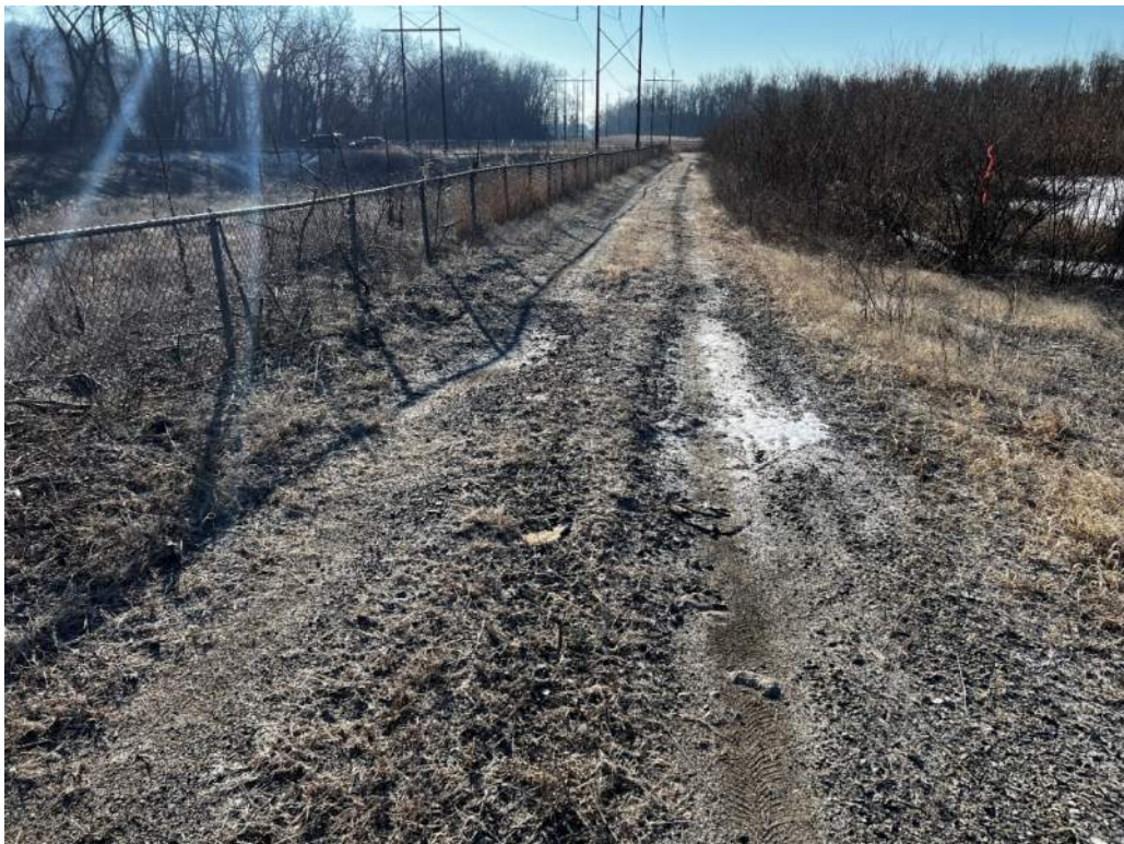
Photo 6 –Low area with rutting on west crest
