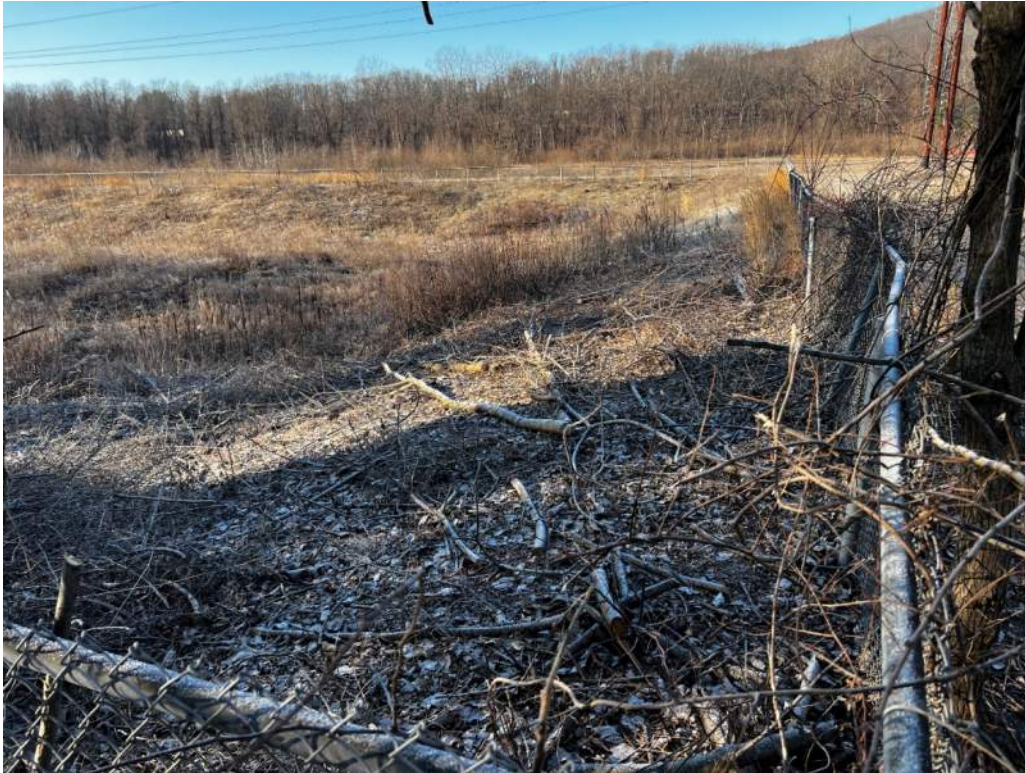
Photo 11 – North embankment interior slope; note cut vegetation
