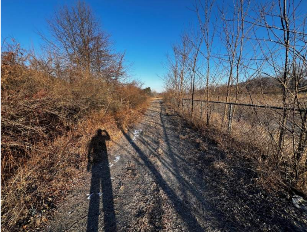
Photo 21 – West embankment looking north; note woody vegetation along interior slope
