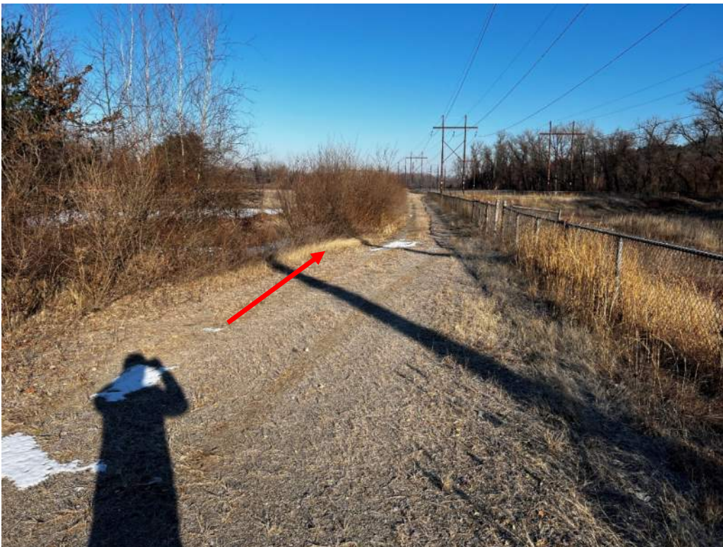
Photo 2 – West embankment crest looking north; note low area (red arrow)
