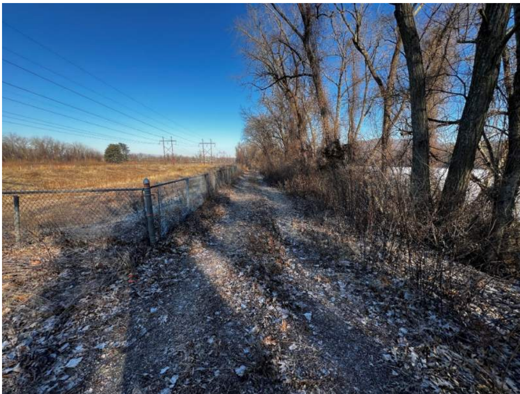
Photo 20 –East crest; note trees on exterior slope
