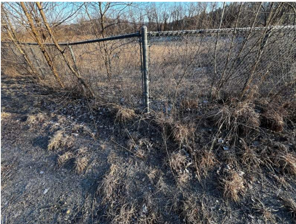
Photo 20 – Bending of fence section, potentially due to mechanical contact (e.g., fallen tree or construction equipment)
