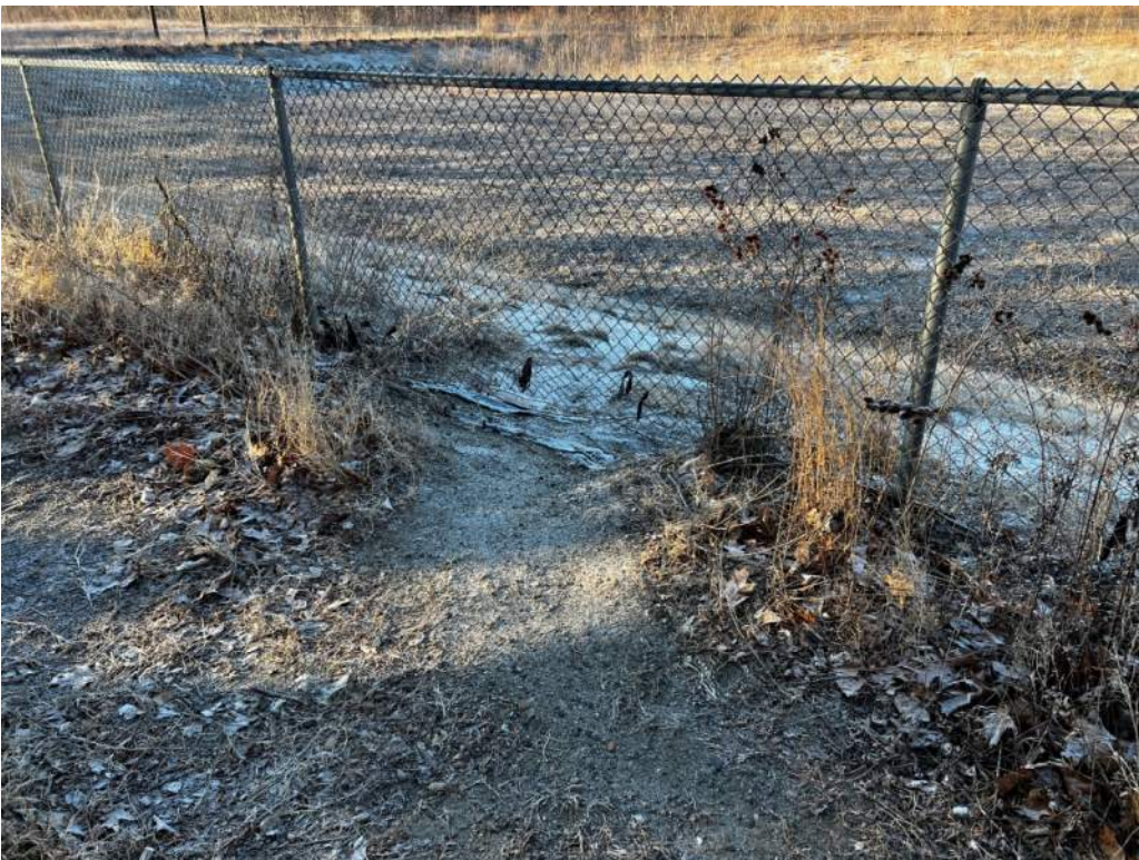
Photo 8 – Low, eroded area at upstream edge of crest on east embankment
