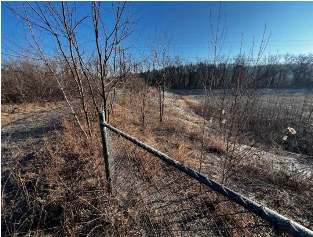
Photo 23 – South interior slope; note woody vegetation and areas of sparse cover
