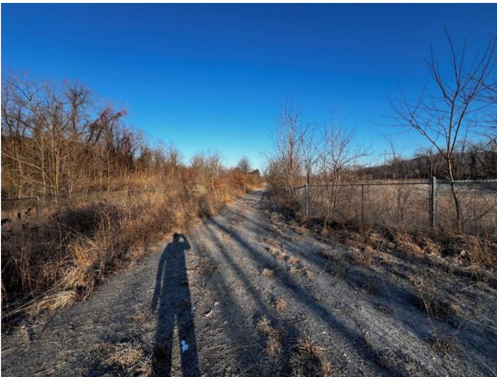
Photo 18 – West embankment looking north; note woody vegetation along interior slope
