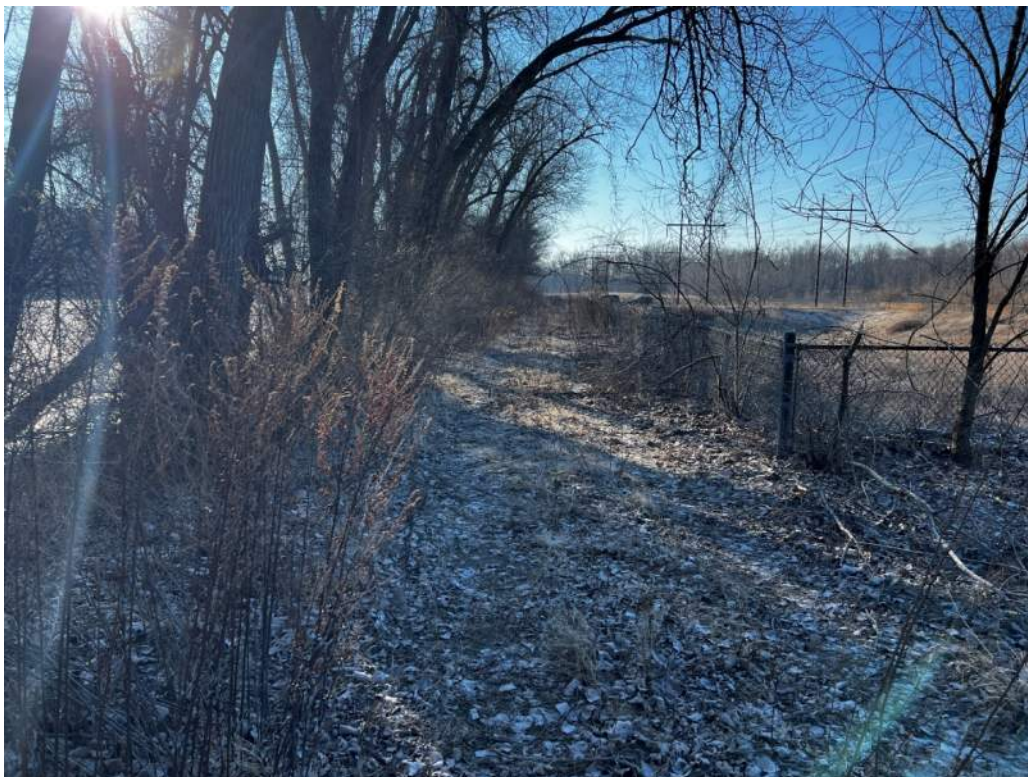
Photo 12 – East embankment crest looking south; note trees on exterior slope and brush growing along fence line.
