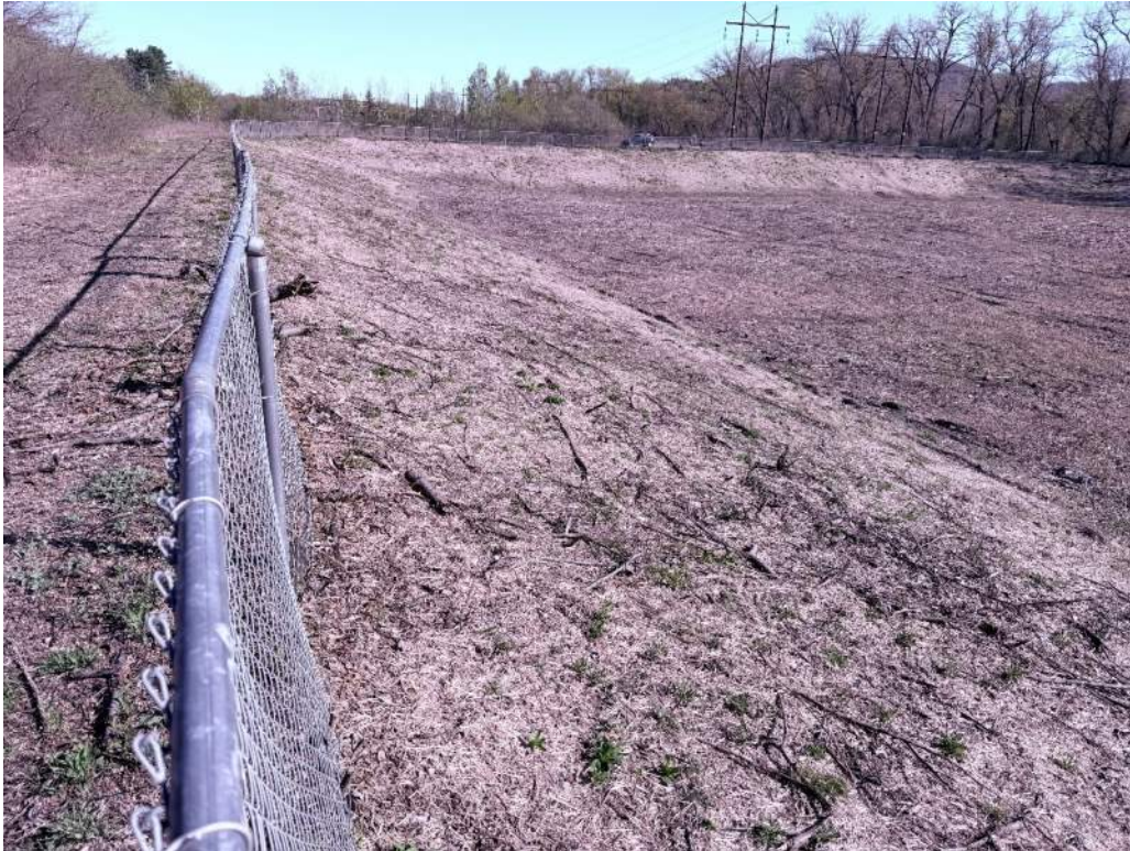
Photo 23 - West interior slope; vegetation remains sparse but slope has been recently seeded and mulched
