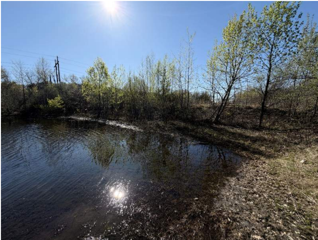
Photo 29 - North exterior slope along coal pile sump; note woody vegetation
