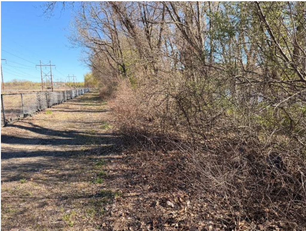
Photo 14 - East exterior slope from south; note heavy trees and brush
