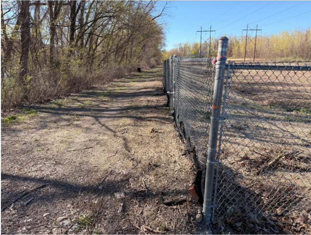
Photo 5 - Berm along top of interior slope
