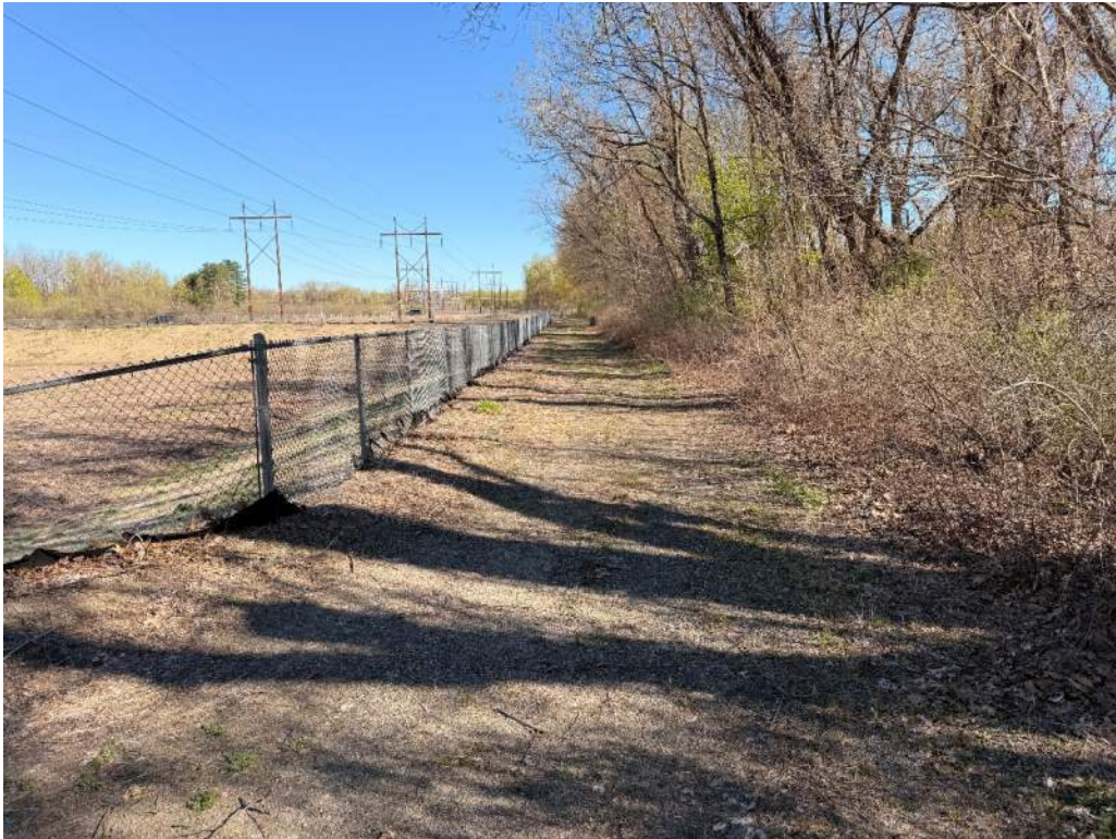
Photo 13 - East embankment crest from south; note marginal vegetation
