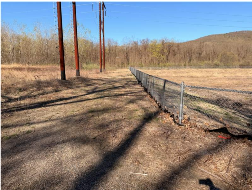
Photo 16 - South embankment crest; area appeared to have been mulched
