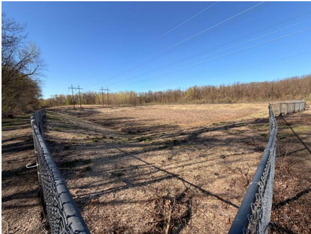
Photo 4 - Interior of basin from northeast corner
