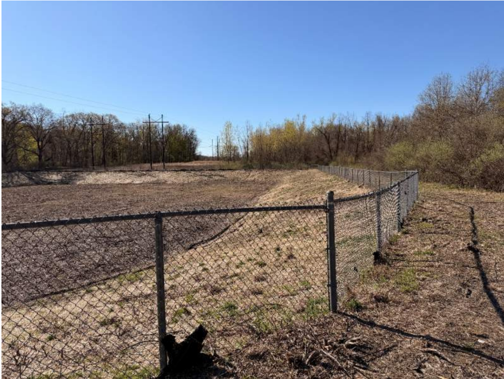
Photo 25 - West interior slope from north; woody vegetation has been removed
