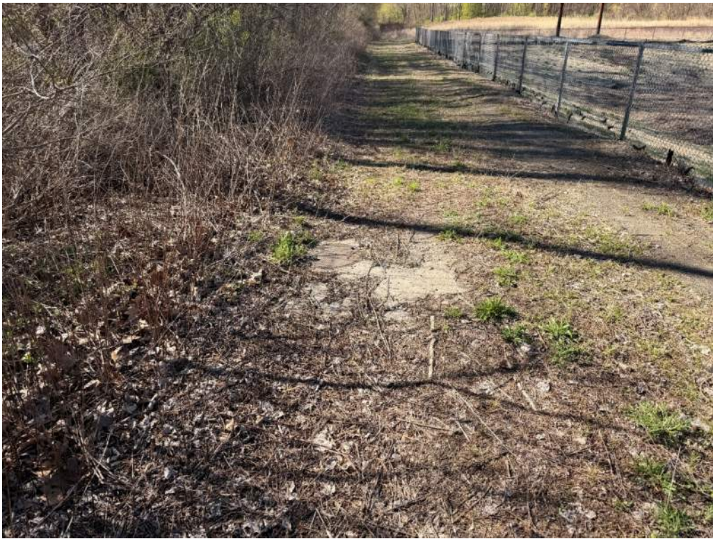
Photo 10 - Access cover along east embankment crest
