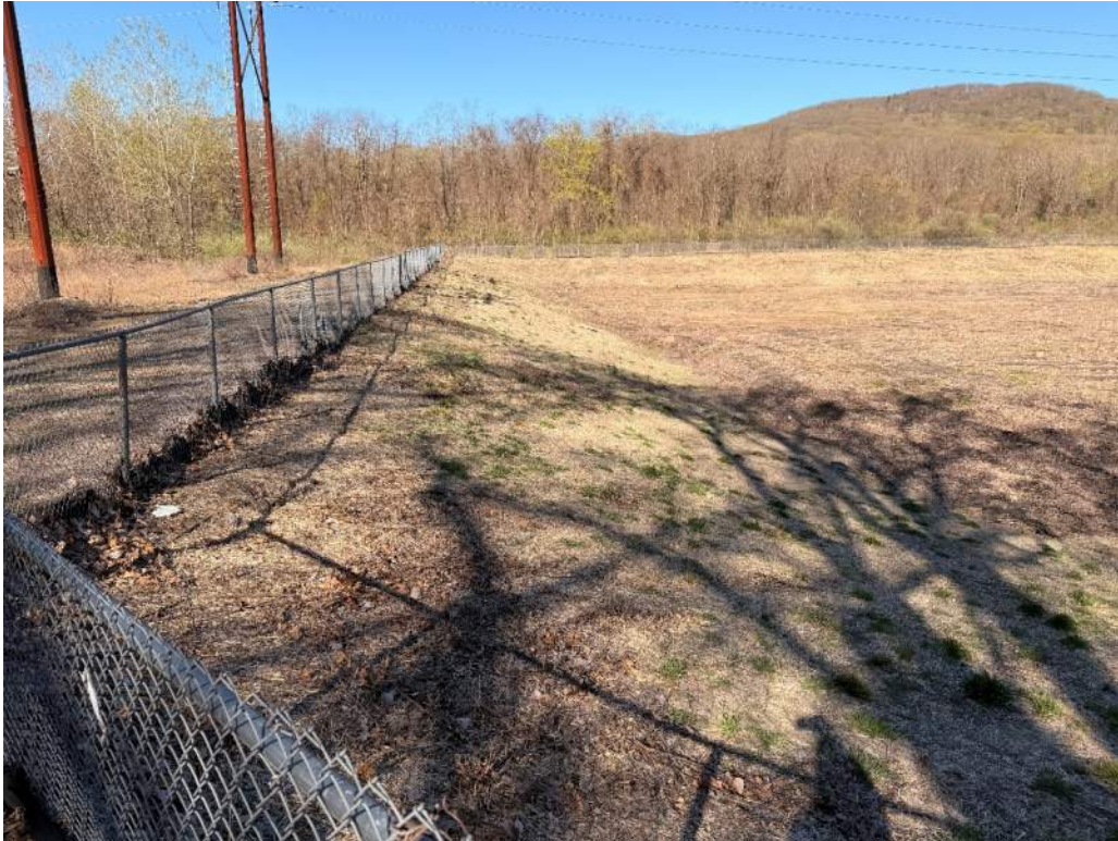
Photo 15 - South interior slope; vegetation remains sparse but slope has been recently seeded and mulched
