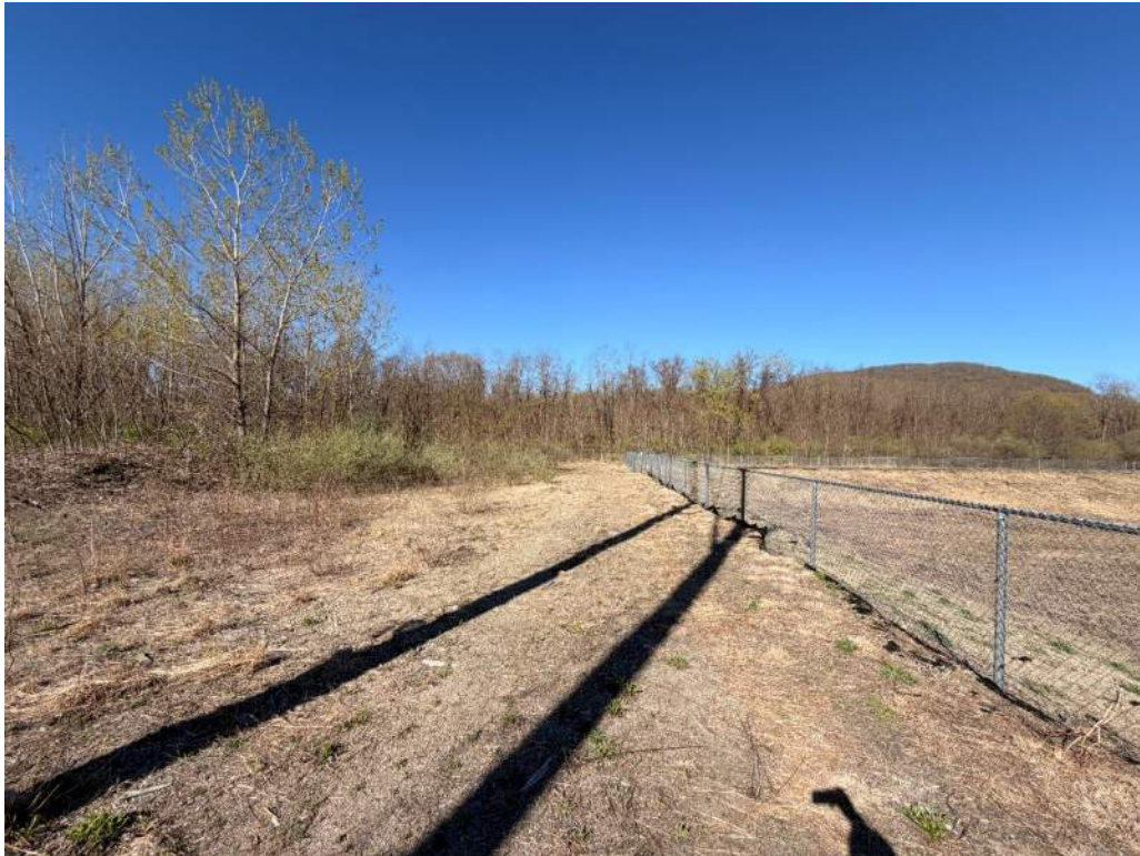
Photo 17 - South embankment crest; area appeared to have been mulched
