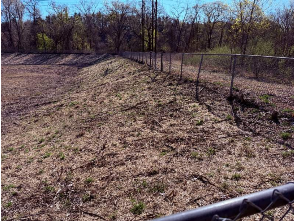
Photo 19 - South interior slope from west looking east; brush along fence line has been cleared
