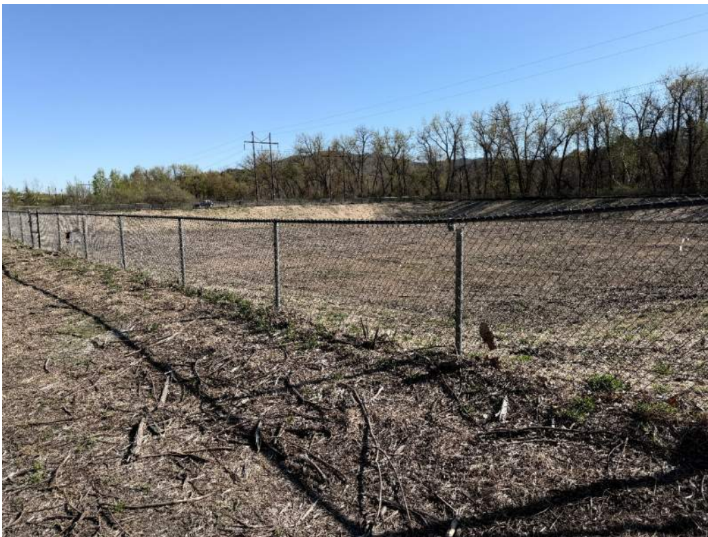
Photo 22 - Repaired section of chain link fence
