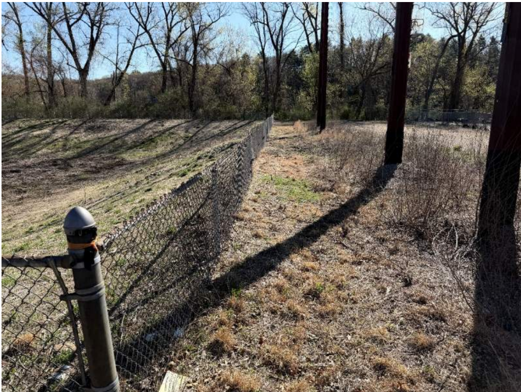
Photo 30 - North exterior slope along Special Basin
