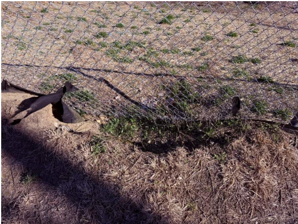
Photo 18 - Erosion along top of south interior slope
