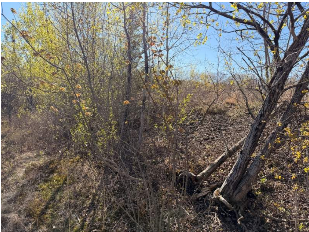
Photo 28 - North exterior slope along coal pile sump; note woody vegetation
