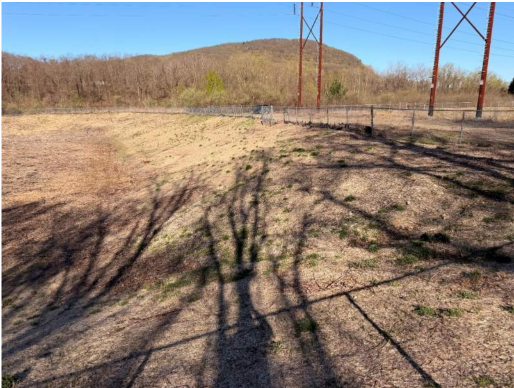
Photo 6 - North interior slope; vegetation remains sparse but area has been seeded and mulched.
