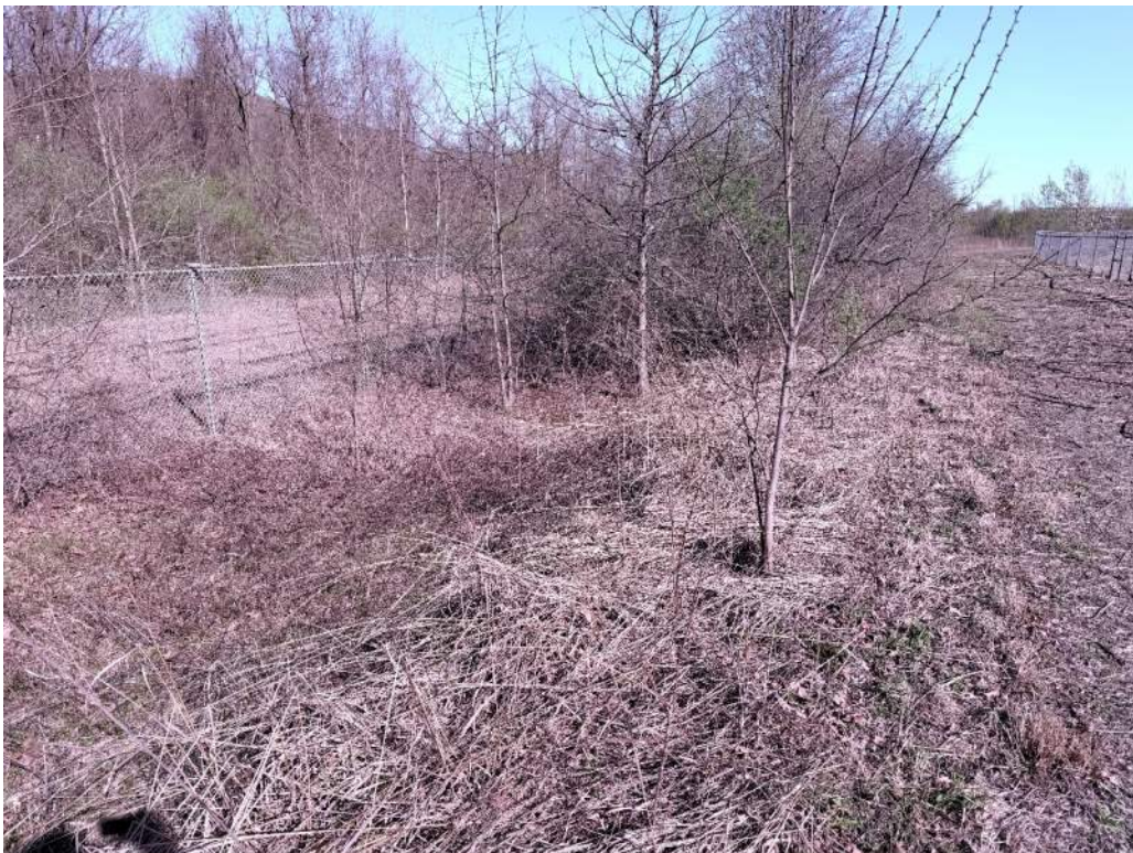
Photo 24 - West exterior slope; note small trees, brush, and woody vegetation
