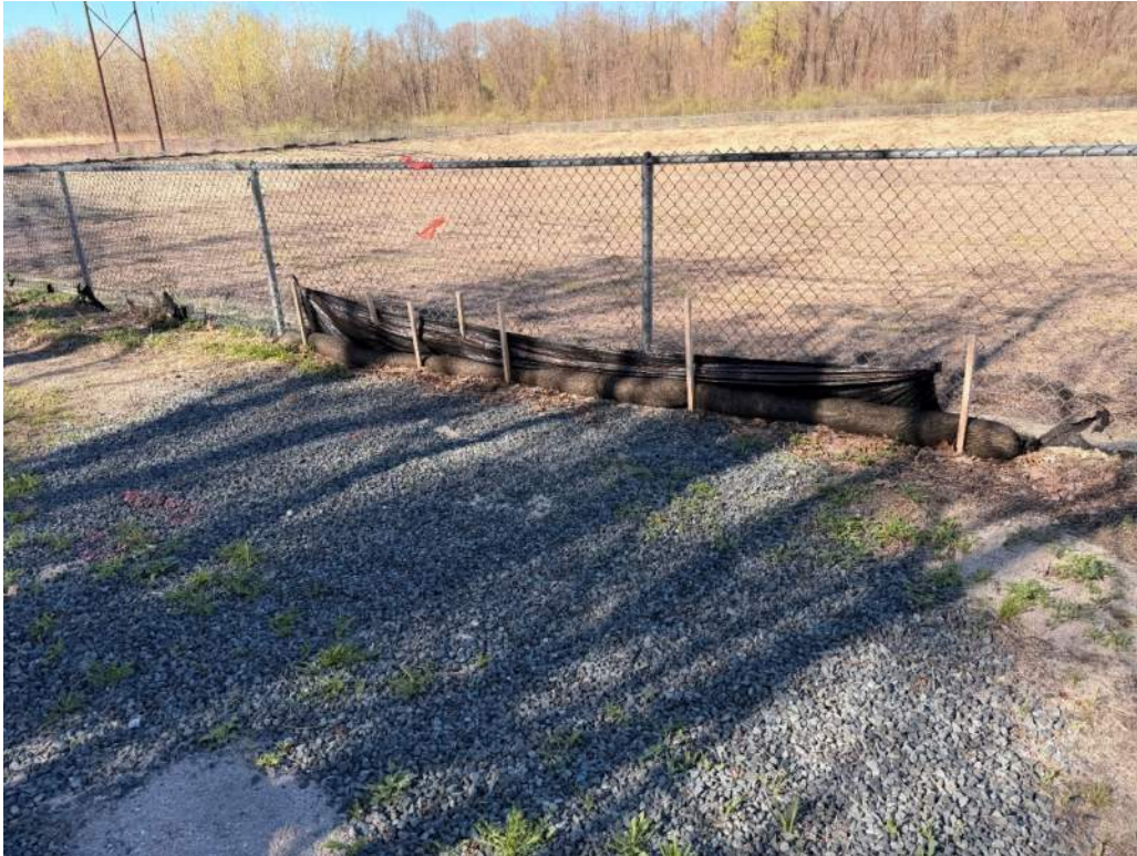
Photo 7 - Repaired area that was previously low and eroded
