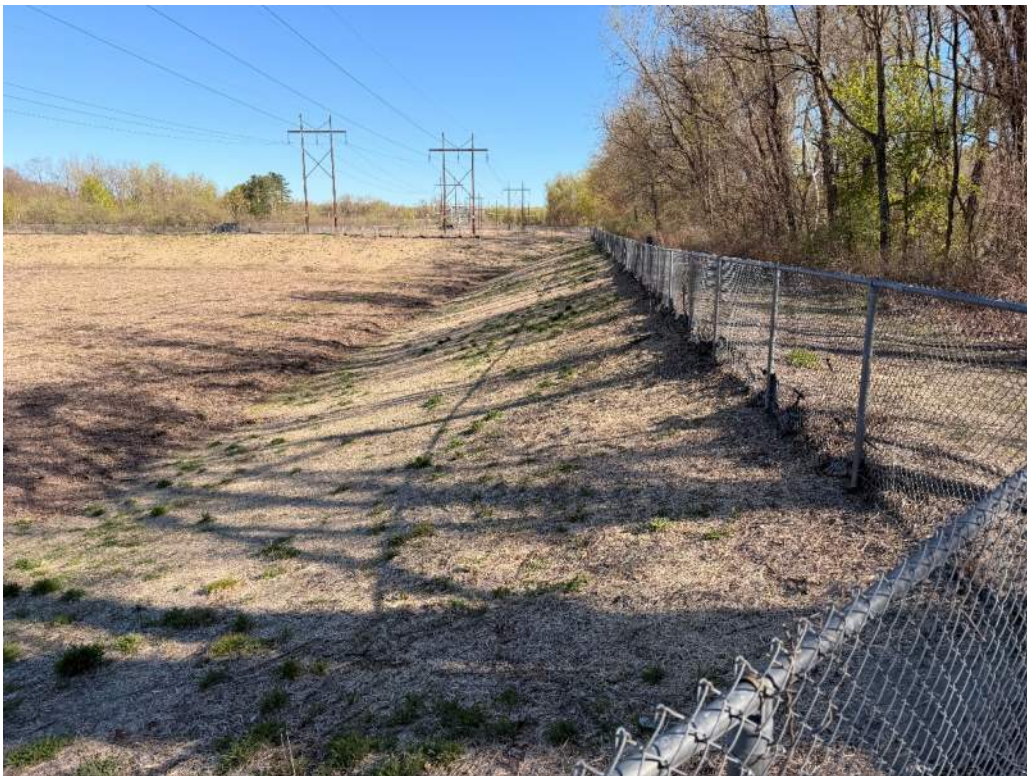
Photo 12 - East interior slope from south; vegetation remains sparse but area has been recently seeded and mulched
