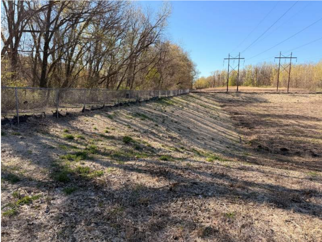
Photo 1 - Bottom Ash Basin A east interior slope; vegetation remains sparse but area has been seeded and mulched
