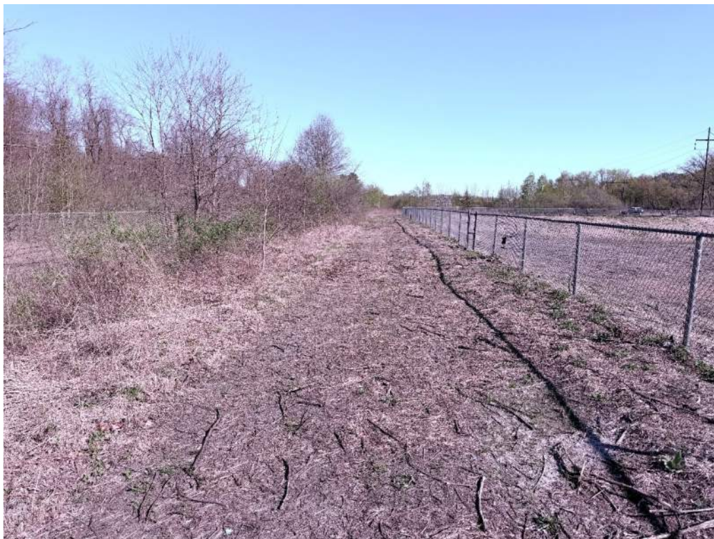
Photo 20 - West embankment crest looking north; brush along fence line has been cleared
