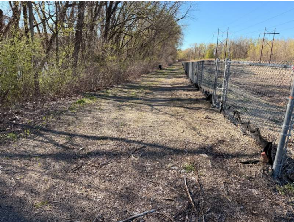
Photo 2 - East embankment crest; note sparse vegetation and minor rutting
