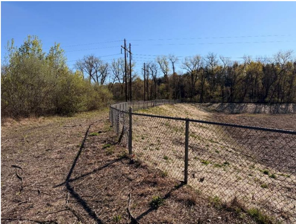
Photo 26 - South interior slope; woody vegetation has been removed; slope has recently been seeded and mulched
